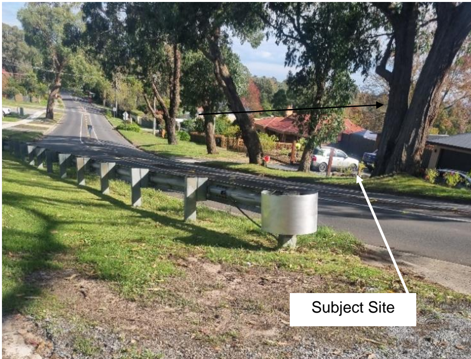
Figure 8 - View along Morris Road looking south.
